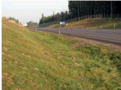
**Figure 4.22. Recoverable fill slope; bottom of the ditch is rounded, no hazardous obstacles in fill slope. (Photo, HUT)**
